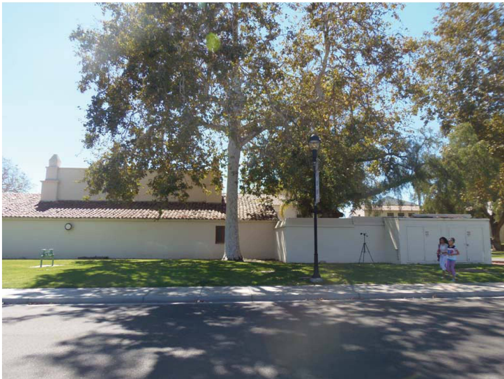
Photo 4: Project site from Camarillo Street.
