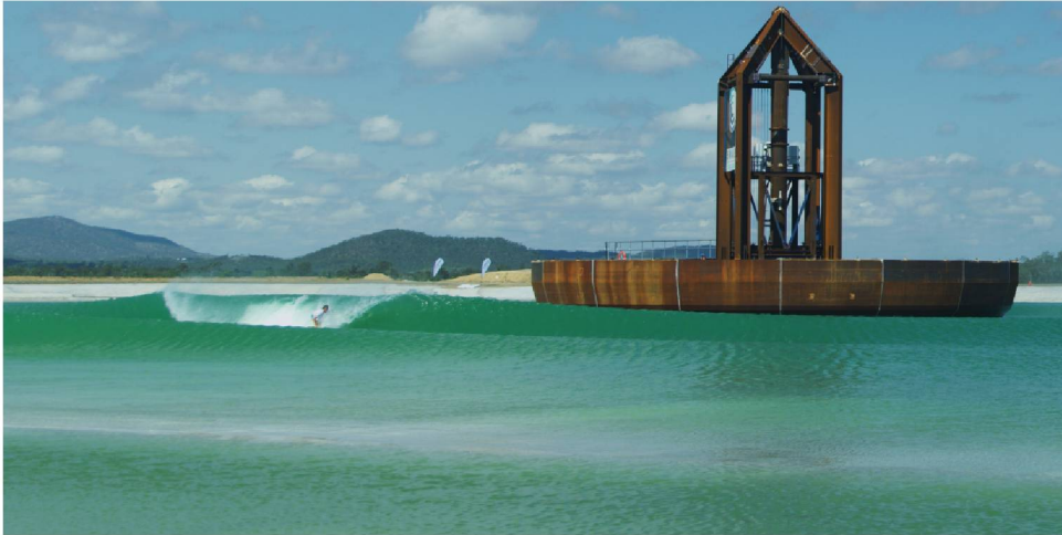
Figure 7.1: This is a wave pool in Australia that uses the "plunger" in the middle and compressed air to generate waves.
